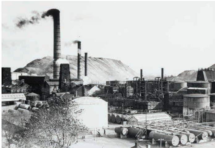
Pumpherton Oil Works: The scale of the operation is clear. MUSEUM OF THE SCOTTISH SHALE OIL INDUSTRY
